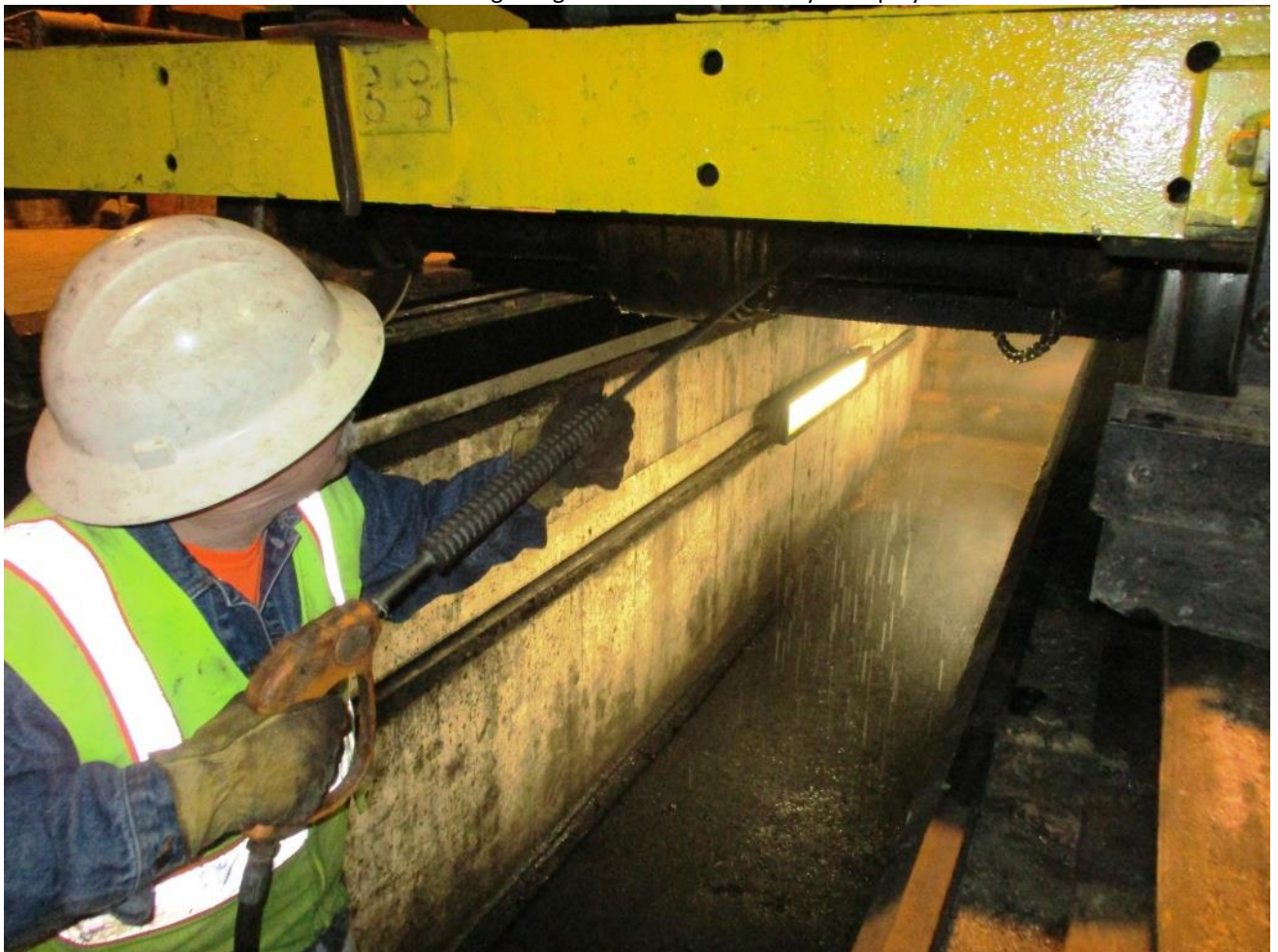
Mike H. steam-cleans the underside of the Kalamazoo so that the turntable can be welded-up
