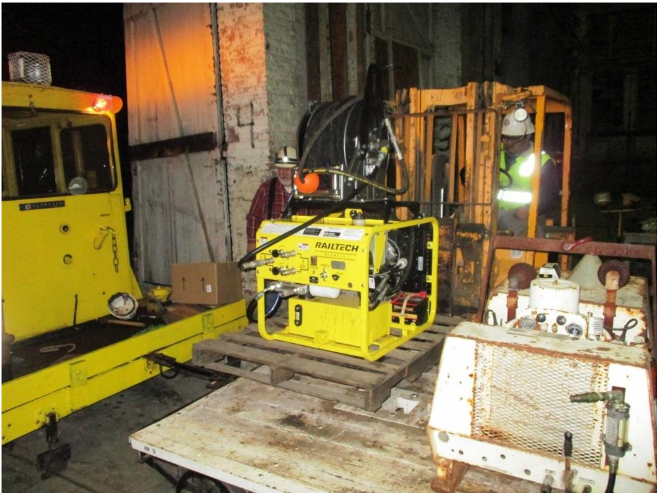
Anthony loads the new hydraulic power unit onto the flatcar behind the Kalamazoo
