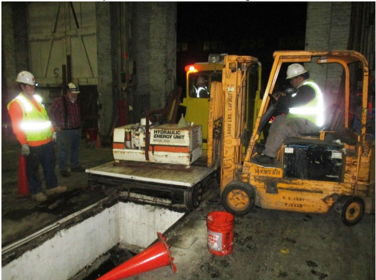
Anthony on the forklift loads the new-used hydraulic power unit on the flatcar guided by Chris H. and Frank
