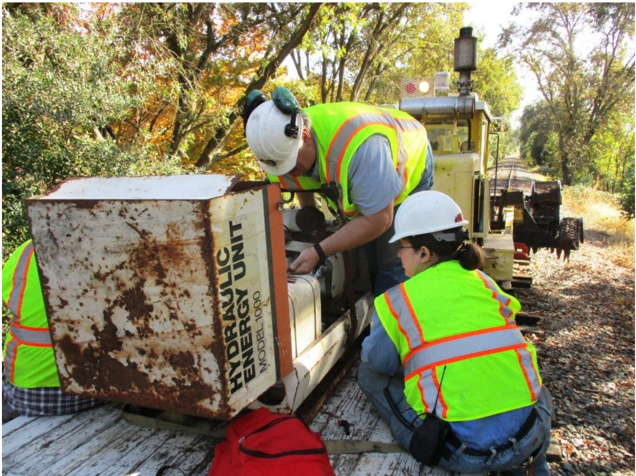
Chris and Heather work on getting the used hydraulic power unit started again after it quit
