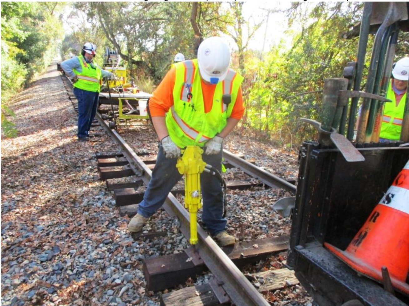
Chris H. finally learns that hydraulically-powered spike-driving is much easier than doing by hand
