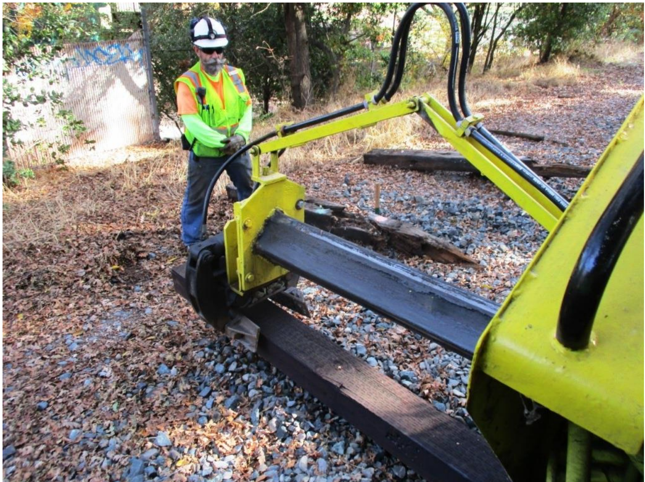
A tie under a joint needed replacing, so Joe lined up a new tie for insertion as the Jackson 125 pulls it under the rails
