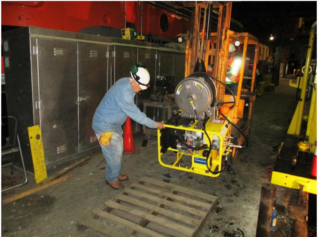
Mike W. guides Ed on the forklift as the hydraulic power unit is loaded onto a pallet
