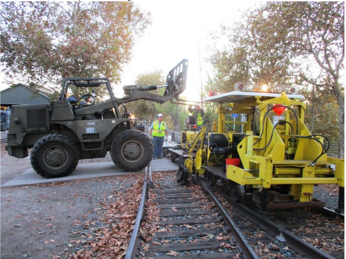
Since GM2 was still in Old Sac., Steve uses it to unload the hydraulic power units from the flatcar
