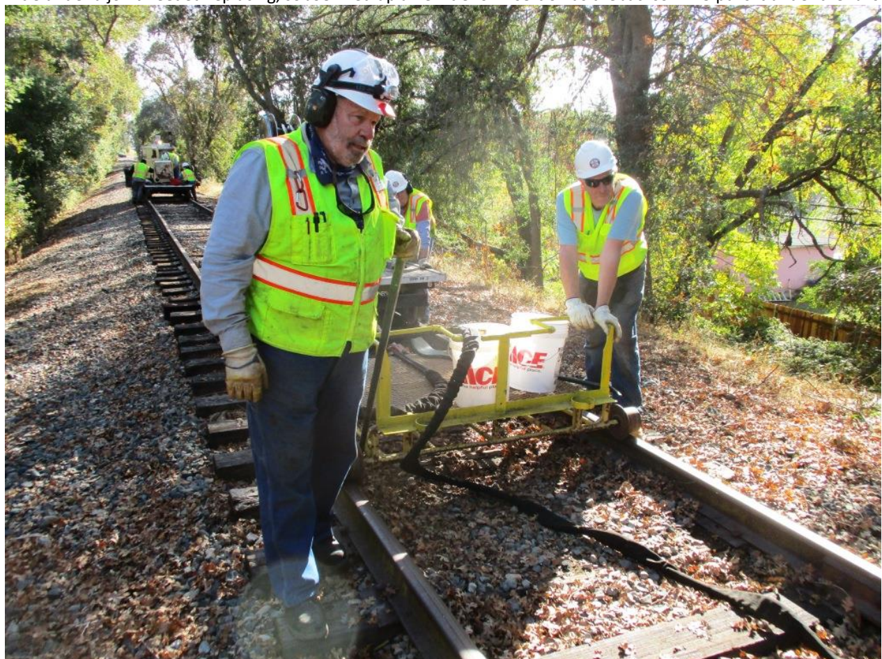
Art and Scott pull the Nolan Track Cart along behind the spiking action
