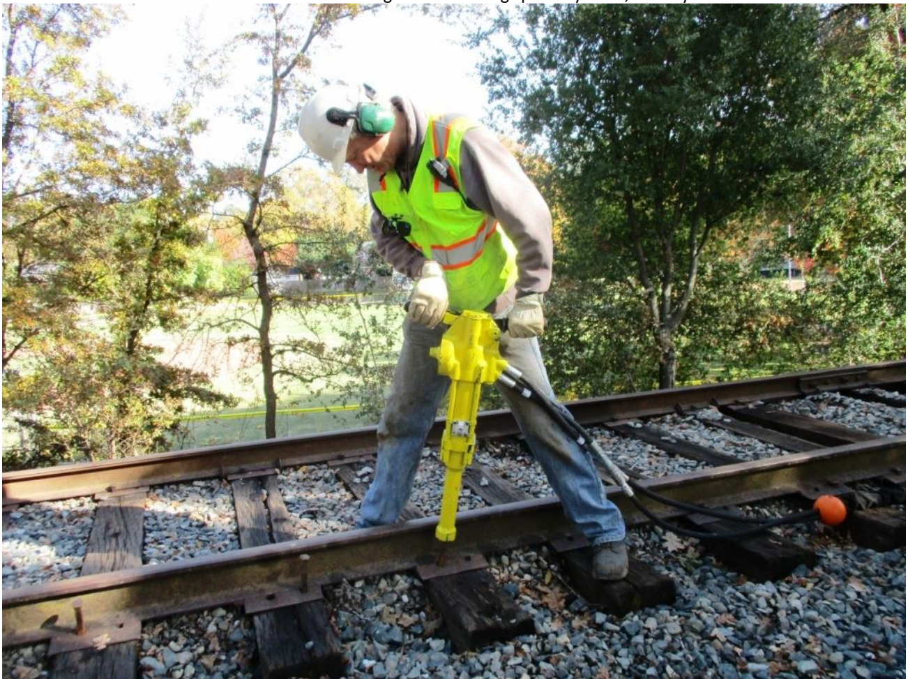
Steve N. demonstrates the proper way to drive spikes – with hydraulic power
