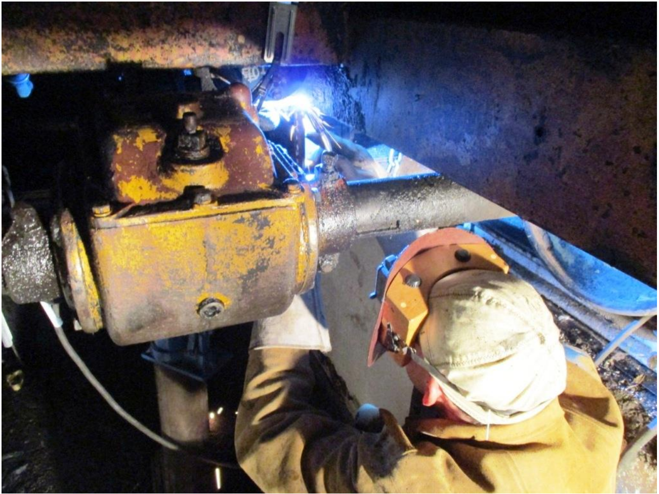
Cliff welds-up the Kalamazoo's turntable
