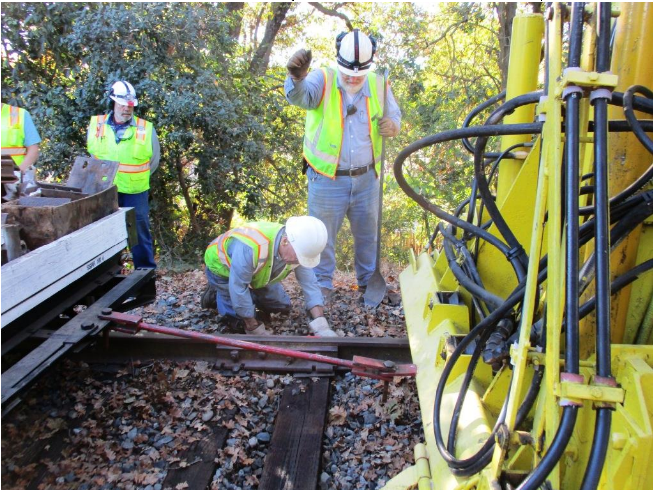
Now Mike T. places a joint-plate under a joint as Frank guides the lift by Chris C. in the 125
