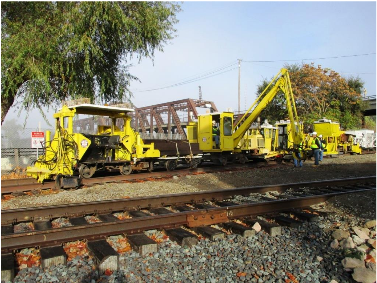
The MOW Team's Great Yellow Fleet: the Jackson 125, tie-crane, scarifier must be moved to access the tie-shear
