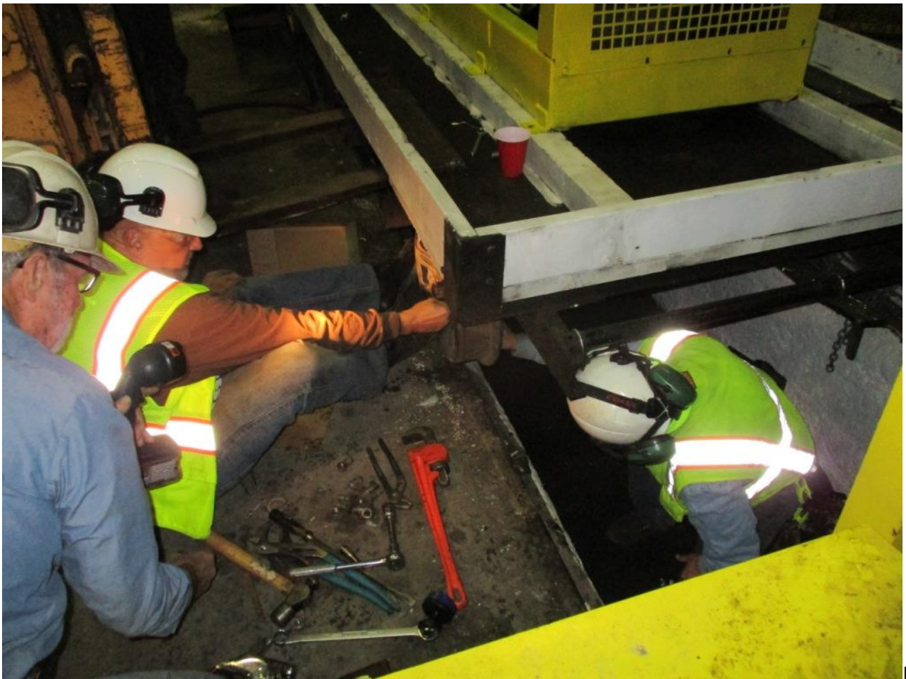
Alan, Dave W., and Joe bolt-down the replacement wheel on the air-compressor's track-cart
