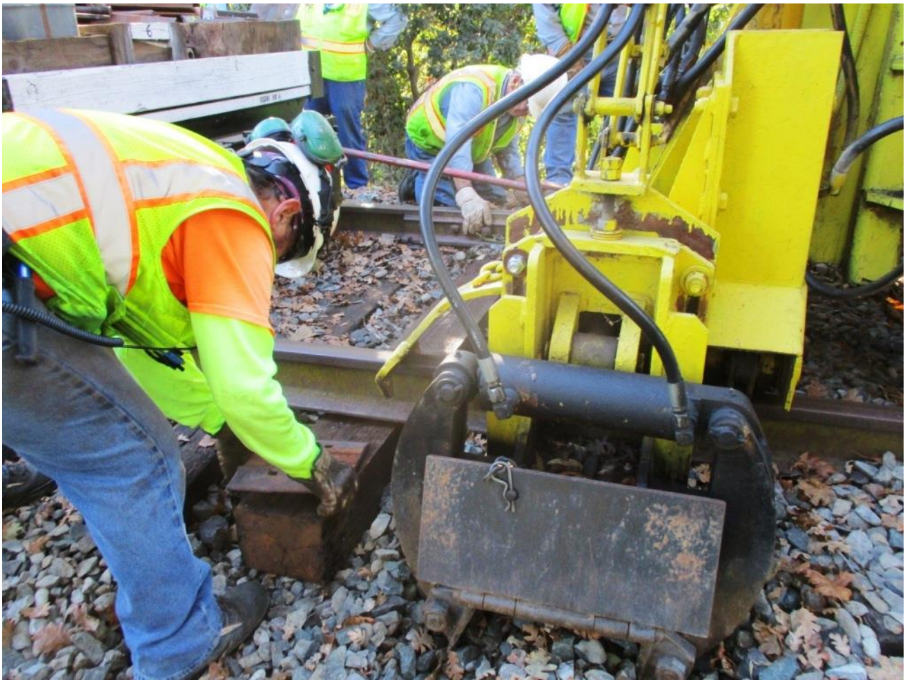
Then Chris uses the Jackson 125's rail-jacks to lift the rail so that Joe can insert a tie-plate
