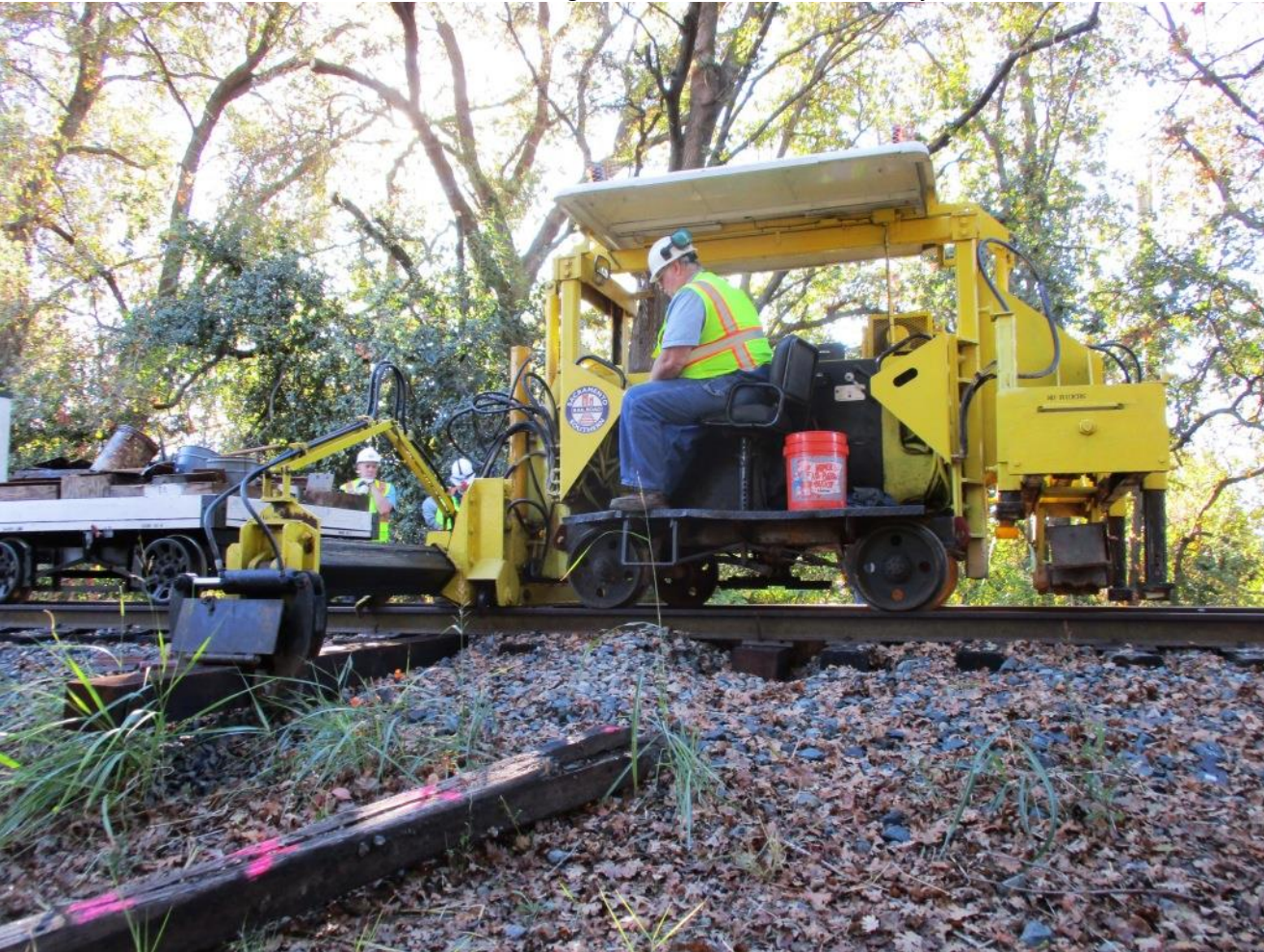
Chris C. uses the Jackson 125 to draw the new tie under the rail
